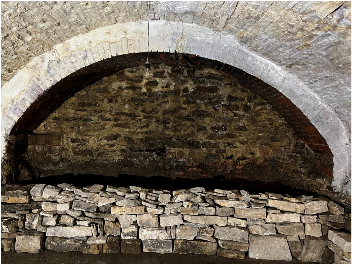
Brick arch at end of boiler room.
