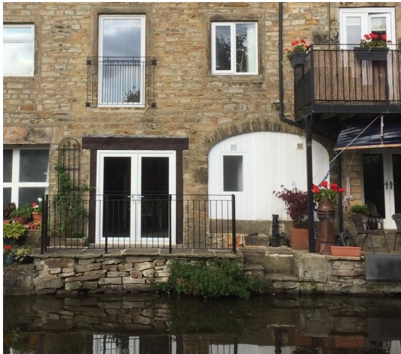
Entrance to the mill coal store from the canal
