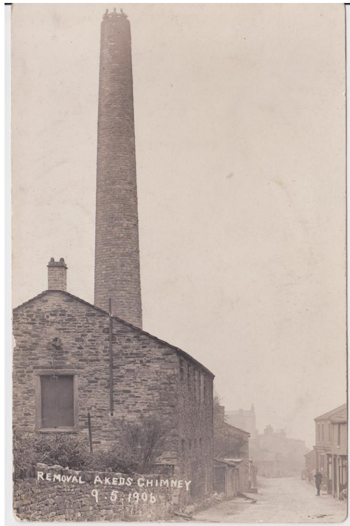
The demolition of Aked's chimney.
