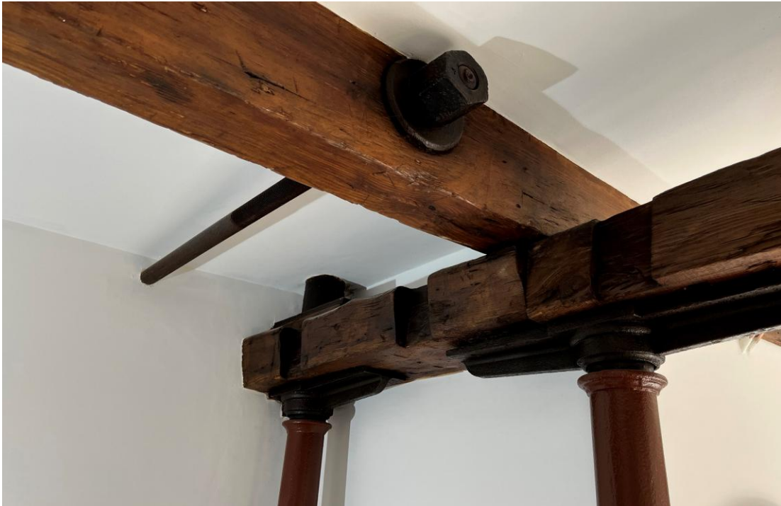
Wooden beams mounted on cast-iron pillars – in the coal store
